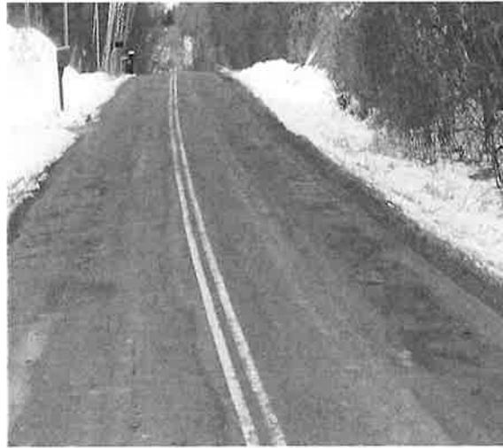
**60<sup>th</sup> Avenue typical Condition showing surface and base failure with rutting and roadway edges breaking off (typical of heavy truck loadings)**
