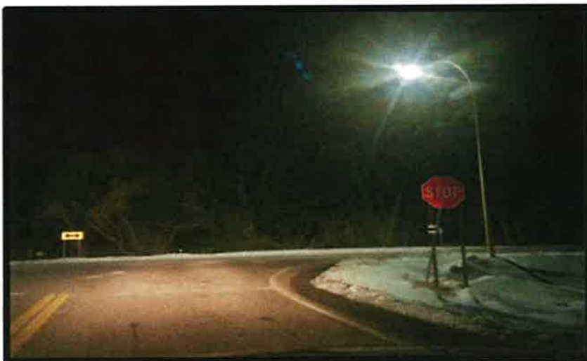
Figure 1 Single overhead light at a rural intersection Source: Minnesota Department of Transportation
